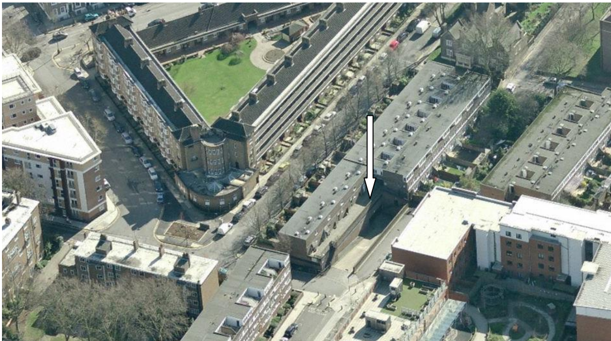
View from Popham Street looking towards the entrance to the site.
